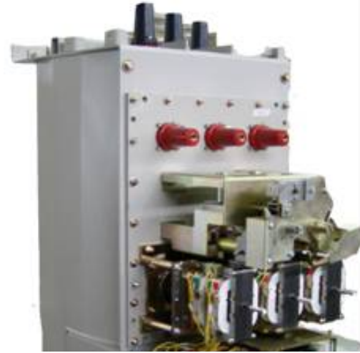
Fig.1. Photograph of the advanced electromagnetically VCB rating 24kV.
