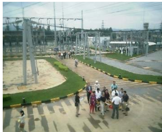
Fig.2 Technical visit (Puji Substation)
