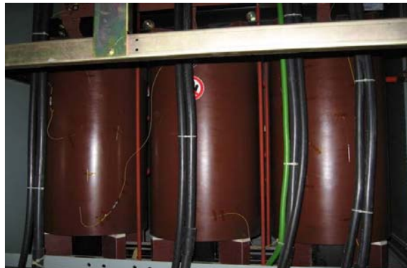
Fig. 1 The 3000kVA mold transformer with the 10 FBG sensors to monitor temperature distributions for 2 months in operation.
