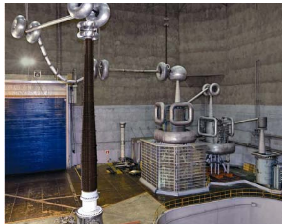
AC withstand voltage test on 1,100kV gas bushing
