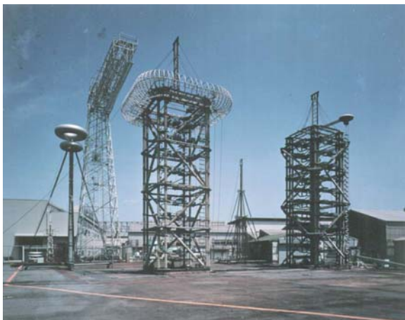
Impulse voltage test facilities
