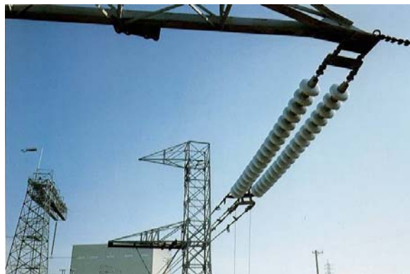
Artificial galloping test of tension insulator assembly
