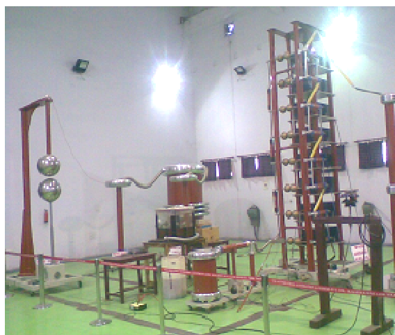
Figure 1: HV Laboratory at NIT, Durgapur
