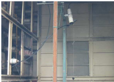
Photo 1. breaking test situation
