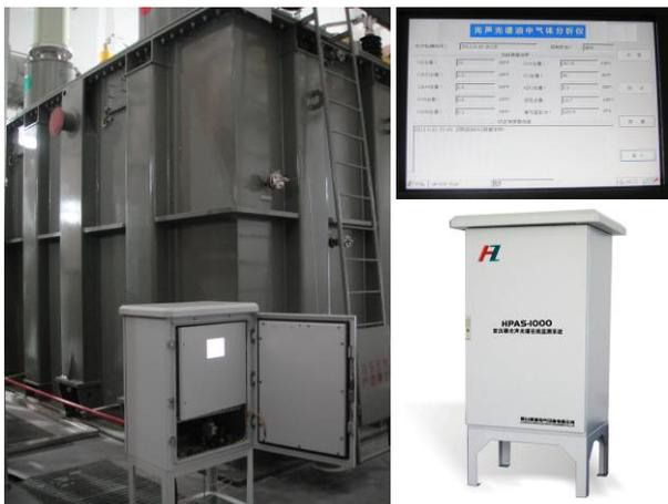
Figure 8. On-line monitoring system for transformer oil dissolved gas (supported by Shanghai Electric Power Corporation)
