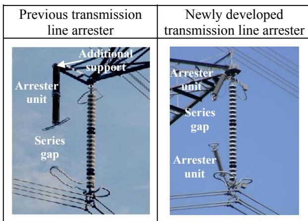
Fig. 1 500kV Transmission Line Arresters
