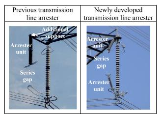
Fig. 1 500kV Transmission Line Arresters
