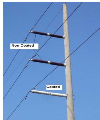
Figure 8 Rod type insulator samples at Ketewel, Bali
