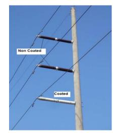
Figure 8 Rod type insulator samples at Ketewel, Bali
