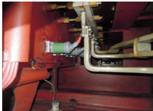
Figure 5 Installed epoxy-mica couplers
