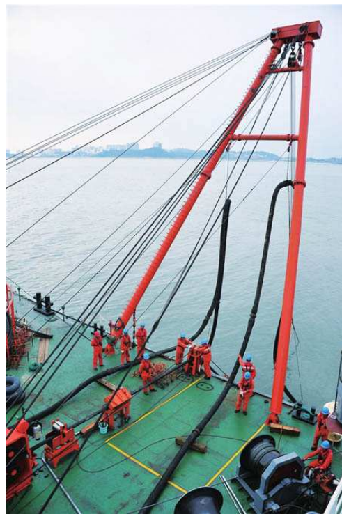
Figure 5. The laying of submarine cable in Nanao three terminal HVDC flexible transmission project
