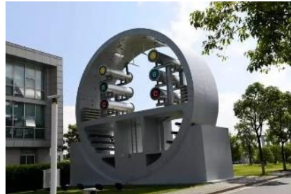
Figure 2. Su-Tong GIL lateral structure and sectional view [2]
