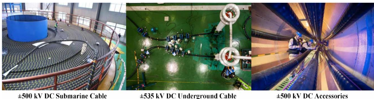
Fig. 1. \pm 500 kV XLPE DC cable and accessories [2-4]
