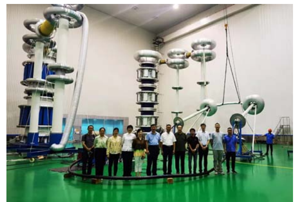
Fig. 5. Witness test site of China's first 110kV thermoplastic PP insulated power cable.
