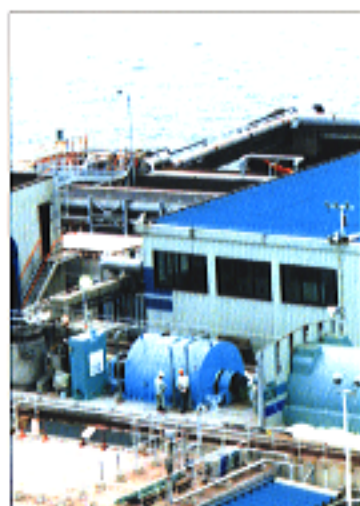
Operational Test of Superconducting Generator
